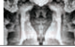
In 2013, Prof. Benjamin Dillenburger and Michael Hansmeyer used a 3D printer to build a 16-square-metre room out of sandstone blocks with details as small as a tenth of a millimetre. They called it “Digital Grotto”
