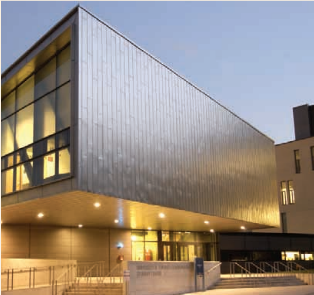
The new student centre at U of T Scarborough includes meeting rooms and lounges for a variety of student organizations and clubs, as well as a prayer room, bookstore, food court and restaurant. Students supported the construction of the environmentally friendly facility with the largest student levy in the university's history.
